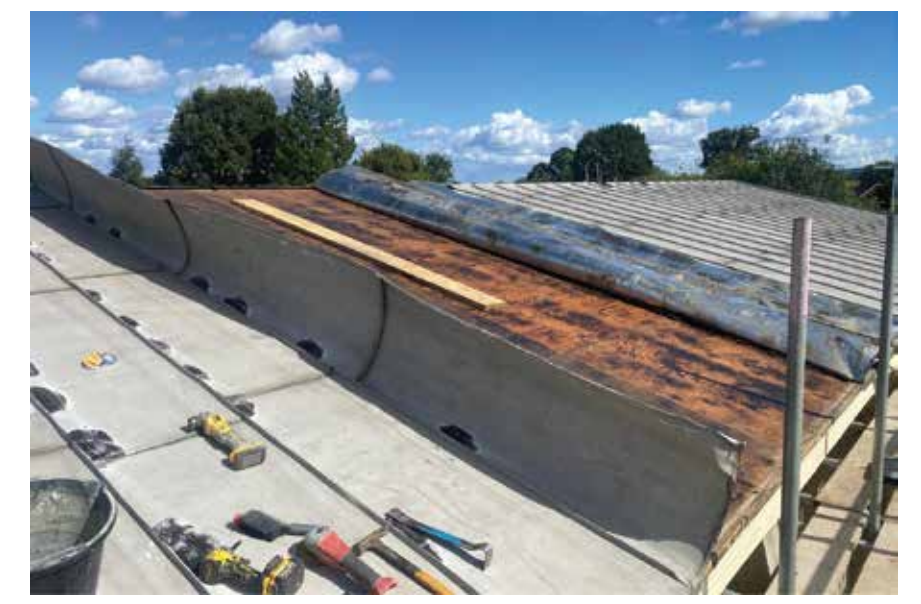
Existing standing seam roofs covered with historic patch repairs
