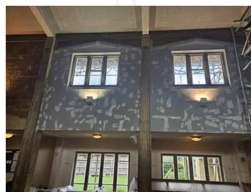
Condition of external walls after injection.
