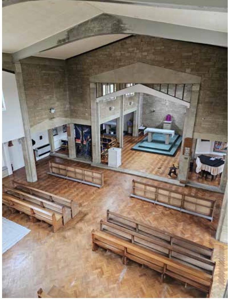
Interior view before renovation.
