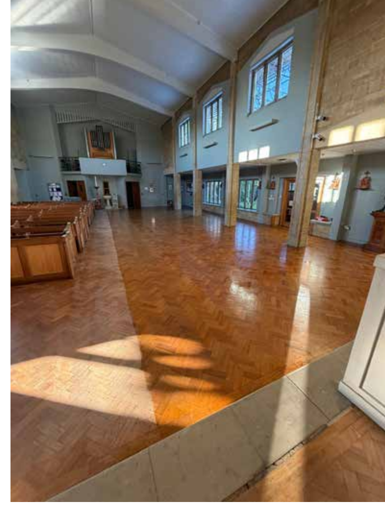
Parquet flooring during renovation.
