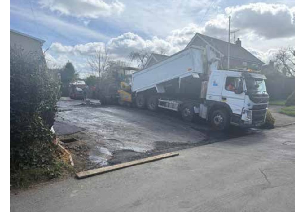
New tarmac surfacing being installed.
