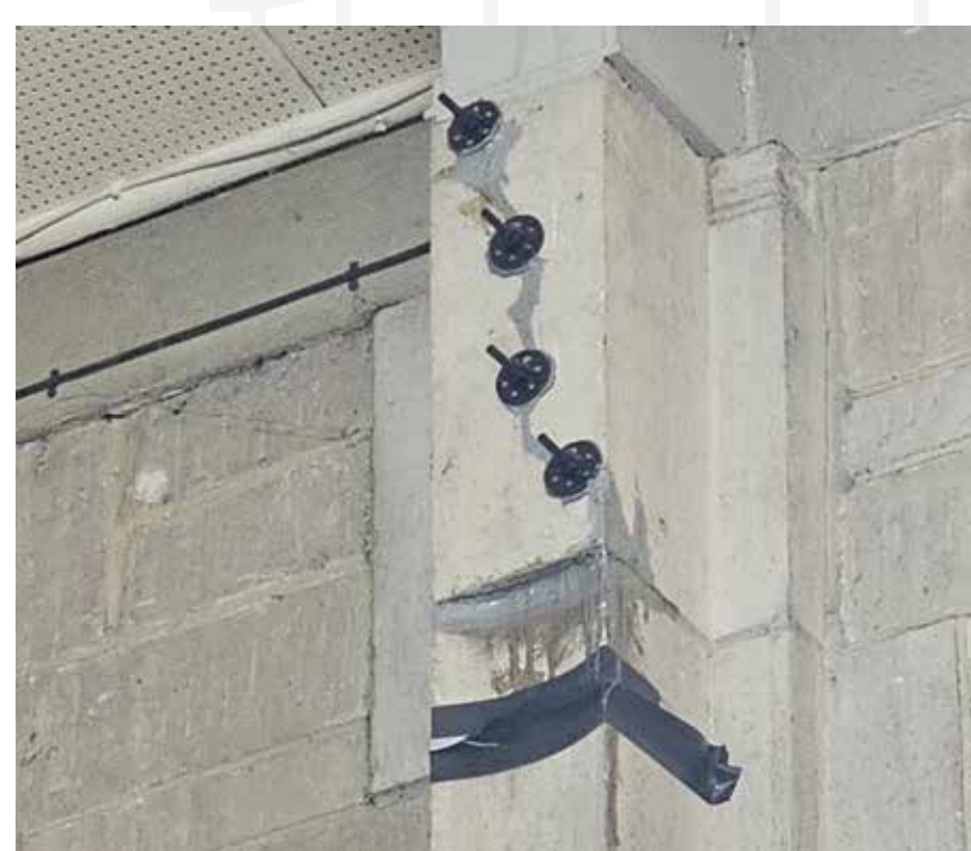
Resin injection of cracks to column.
