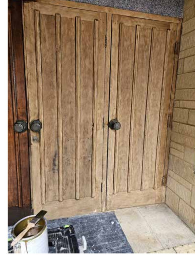
Entrance doors after sanding.
