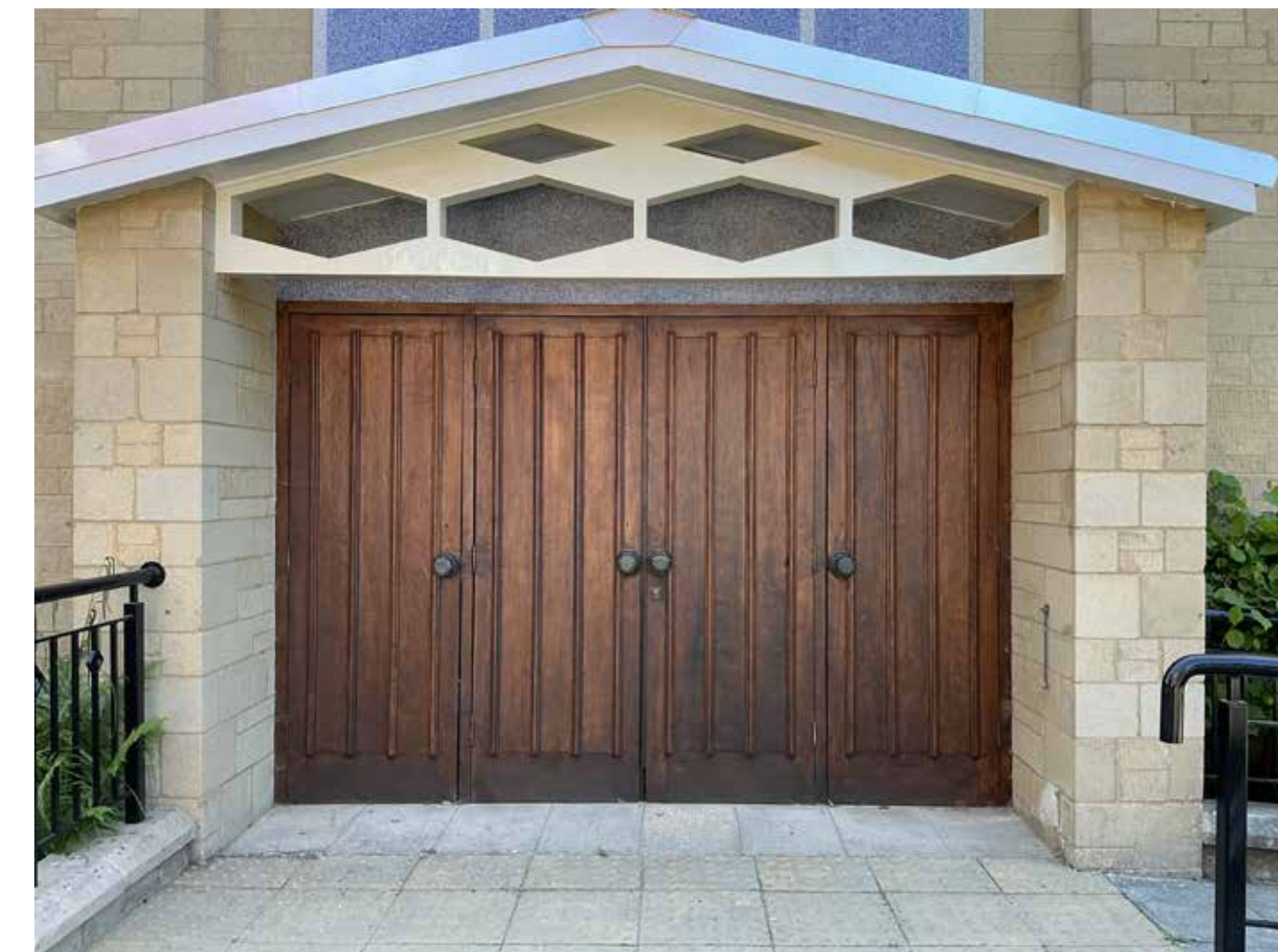
Finished entrance doors after repair, sanding, and staining.
